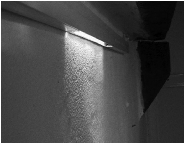
Figure 11-16. Light exit, cut into wire channel
