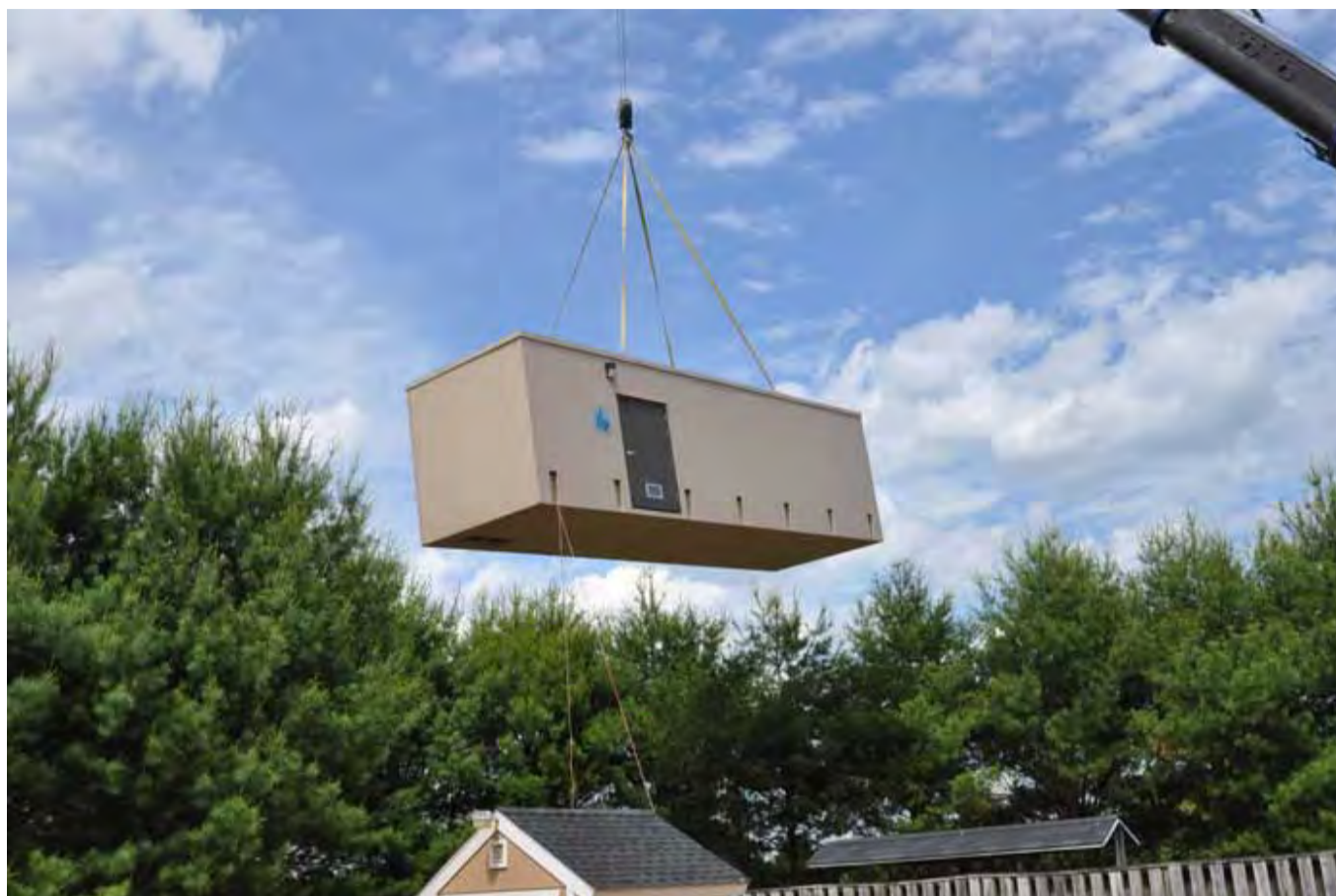
Figure 8K: Single skid ready to run. By starting with a clean slate and avoiding the pitfalls of simply making smaller versions of large plants, new pre-packaged plants using membrane bio-reactor (MBR) technology can operate continuously at 5% of rated capacity, while still delivering high discharge quality in compliance with the highest state and municipal regulations. (Source: ITP)
