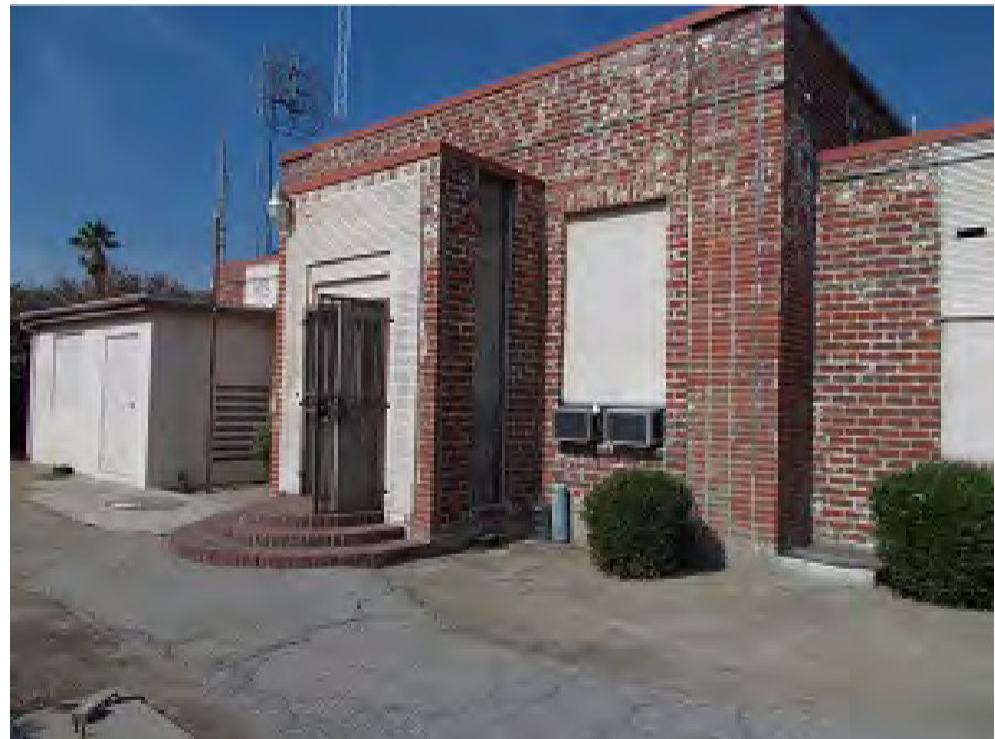
Figure 8A: Many transmitter sites, such as this KLAC radio station facility in Los Angeles, are remote and unattended.
